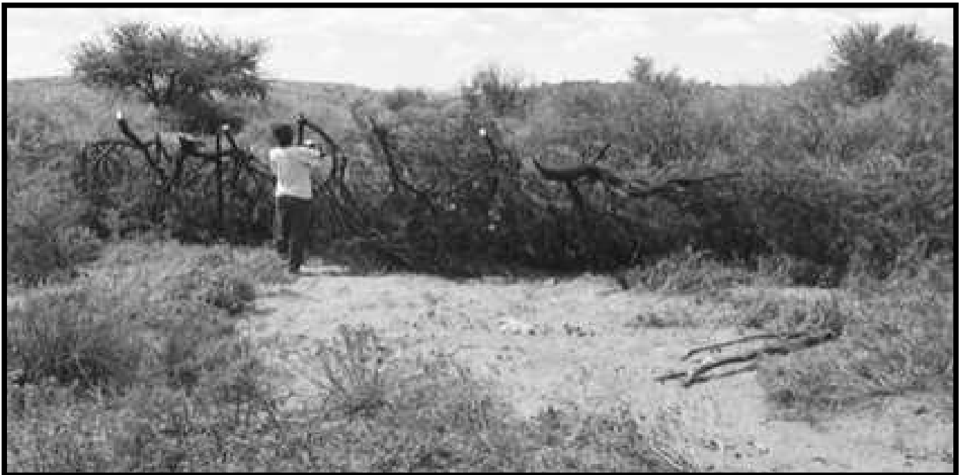
Figure 4. A filter is suspended from wire tied across a gully.
