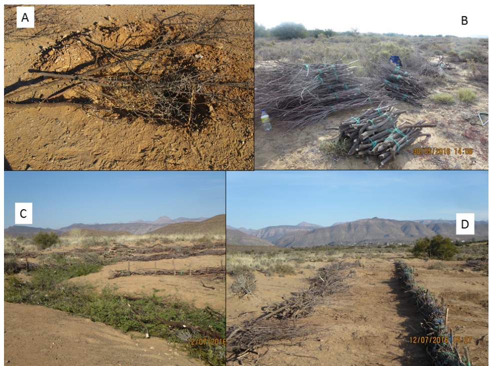
Figure 1. Rehabilitation structures installed at Site 1 in 2016. (A) mulched and brush-covered hollow, (B) materials used, (C) alternating brush-covered hollows and brush fences, (D) brush-packed gullies. (D)
