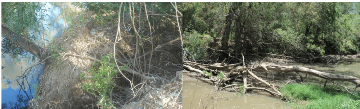
Figure 3: These photos show riverbank erosion due to falling invasive trees in the riparian zone (a) and consequent channel blockage by debris (b), which causes further erosion, in the Berg River in the Western Cape.
