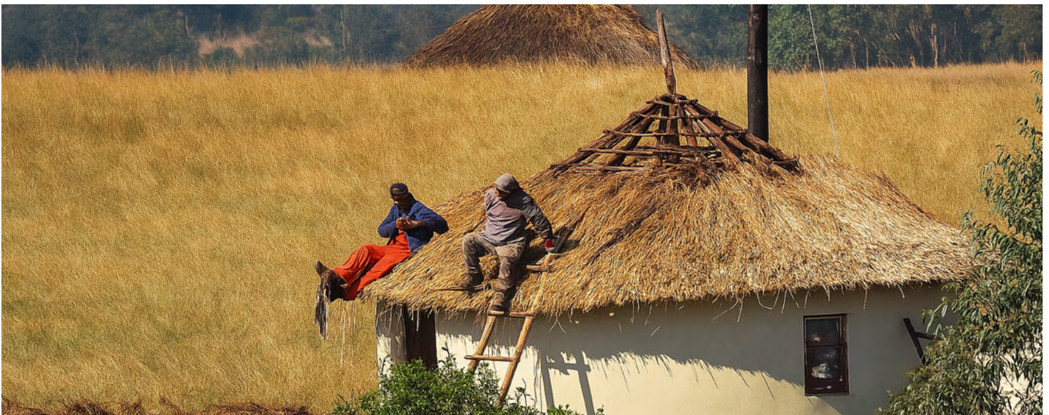
Figure 4. Men at work: Roofing a rondavel with thatch grass.
